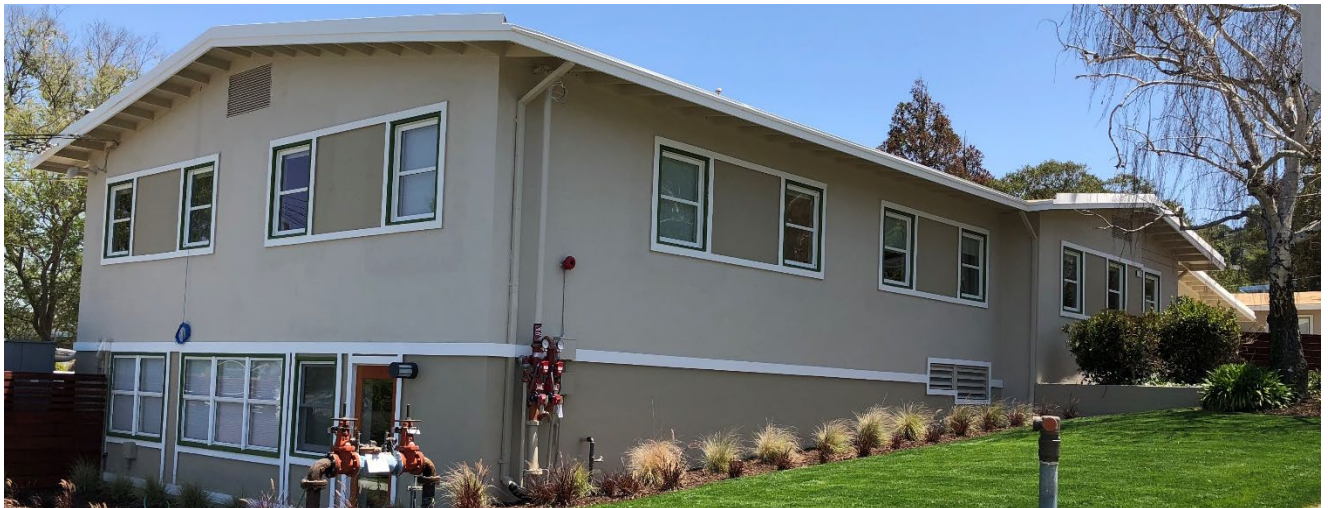
Renovated exterior: Serenity House at Hacienda Street and 37 th Avenue
